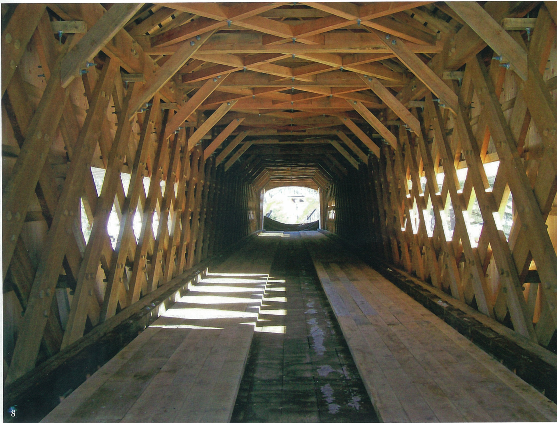
7, 8 New Bartonville bridge, dedicated in January 2013 (despite sign), is 168 ft. long at deck level and 178 ft. overall. Double transverse X-bracing, below, repeats unusual detail of original.
