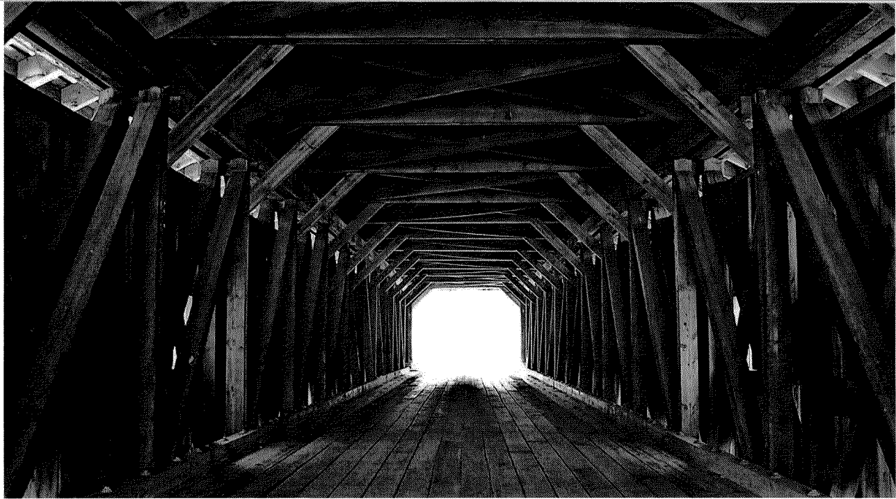
Hamden Bridge, Delaware County, New York, 128-ft.-span Long truss built over Delaware River in 1859 and propped midspan by pier in 1940s. During rehabilitation in 2000, pier was removed and bottom chords replaced by glulam because of theoretical weakness of chord splices, even if in good condition, in original design.
